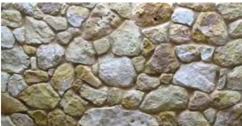
Savings Bank of SA building, and restoration work on St Francis Xavier feature Waikerie Limestone
