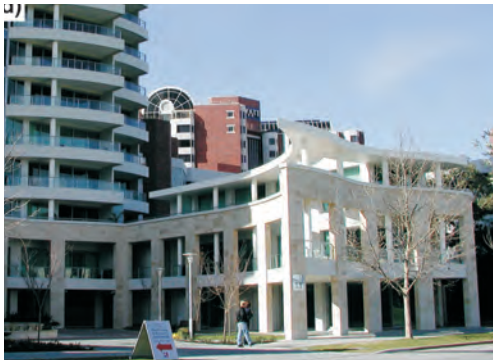
1 Star City, Pyrmont NSW. 2. Donnybrook Sandstone wall framing the entrance to Reconciliation Place, Canberra. 2. contemporary building design in Perth employing pale beige Donnybrook Sandstone cladding
